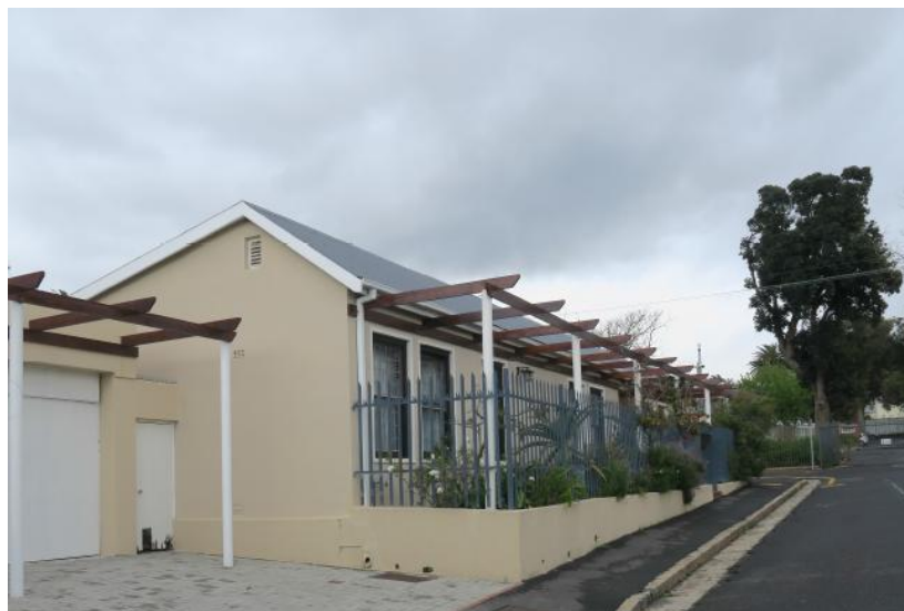
Examples of buildings with heritage significance and active or responsive street interfaces which contribute to the quality of the public environment. Visibility maintained and surveillance improved.
